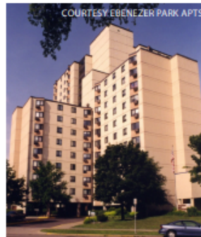
Ebenezer Park Apartments
