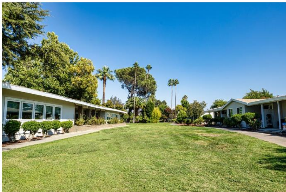
Each apartment unit took about two days to retrofit and residents were able to remain in their units without moving out. Photo by Steve Martarano
