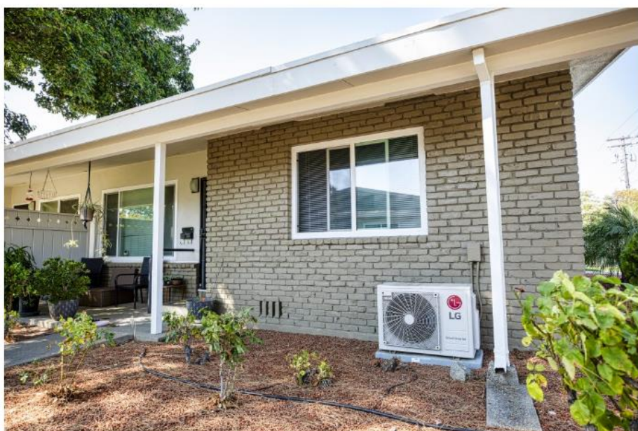
Each retrofit included a total HVAC replacement and new LED lighting. Low-flow shower heads and aerators to reduce water use were installed and refrigerators and windows were replaced as well. Photo by Steve Martarano
