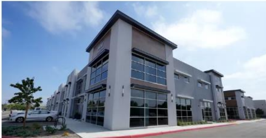
The new Santiago Industrial Suites development in Oxnard put 24 industrial condominiums on a formerly vacant lot at Graves Avenue and Santiago Court, seen Thursday. JUAN CARLO/THE STAR
